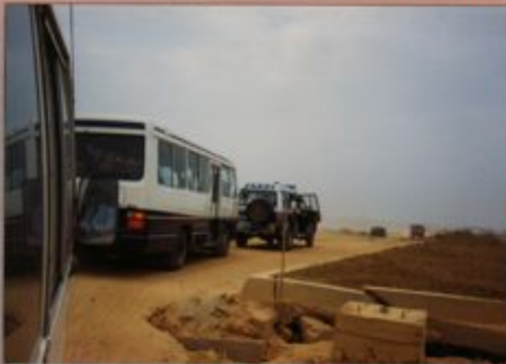
NEW ROAD CONSTRUCTION TO SEAPORT
