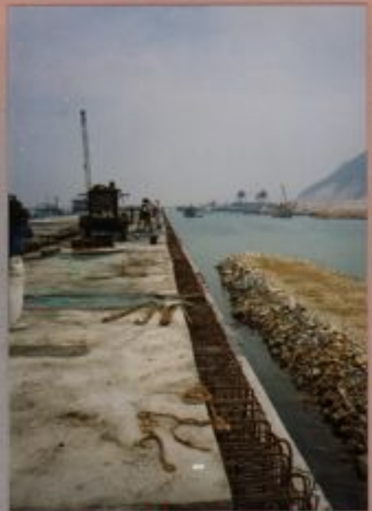
WORK PROCEEDING ON DOCKS
