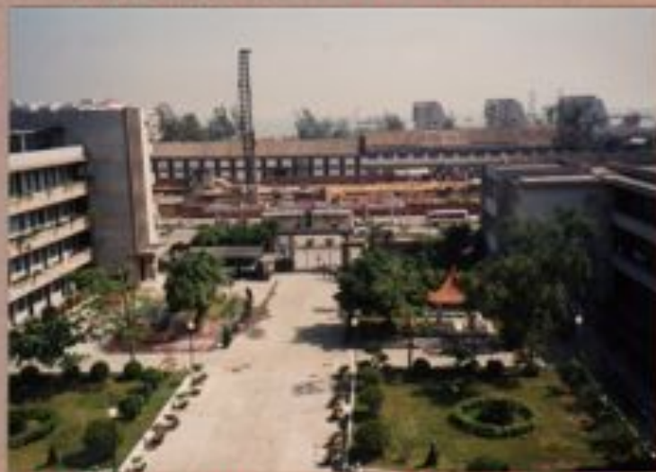
SCHOOL ENTRANCE - NOTE CONSTRUCTION IN BACKGROUND
