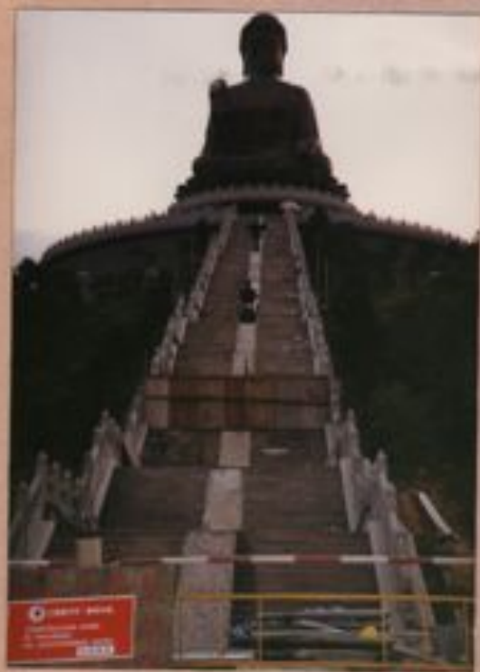
CONSTRUCTION WORK IN PRO- GRESS
