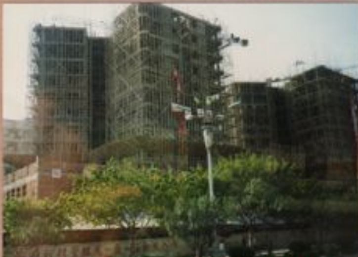
HIGH RISE BUILDING - BAMBOO SCAFFOLD
